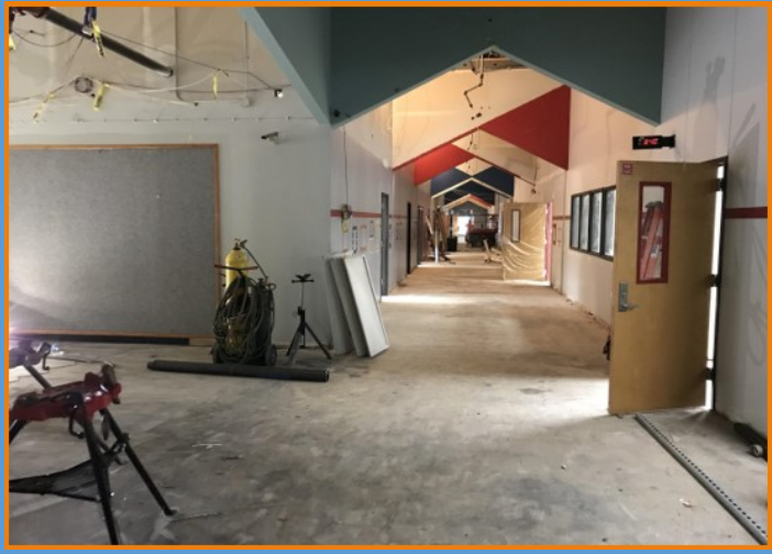
Haun Elementary School, Main Street Demo, July 2019
