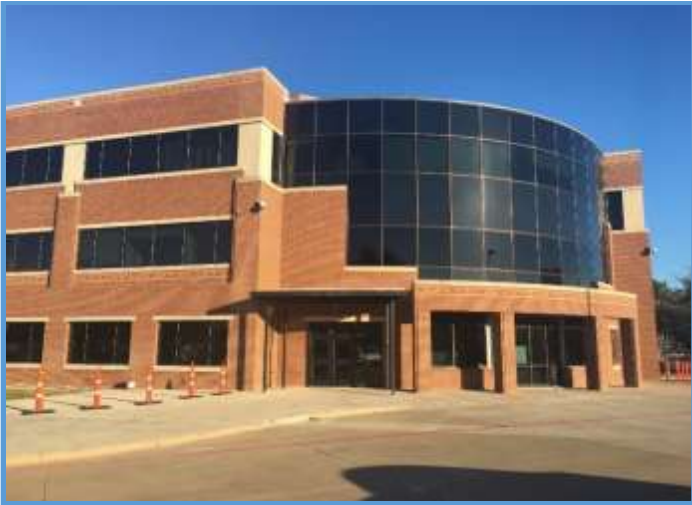
Academy High School Re-Brick, New Brick at West Elevation, October 2017
