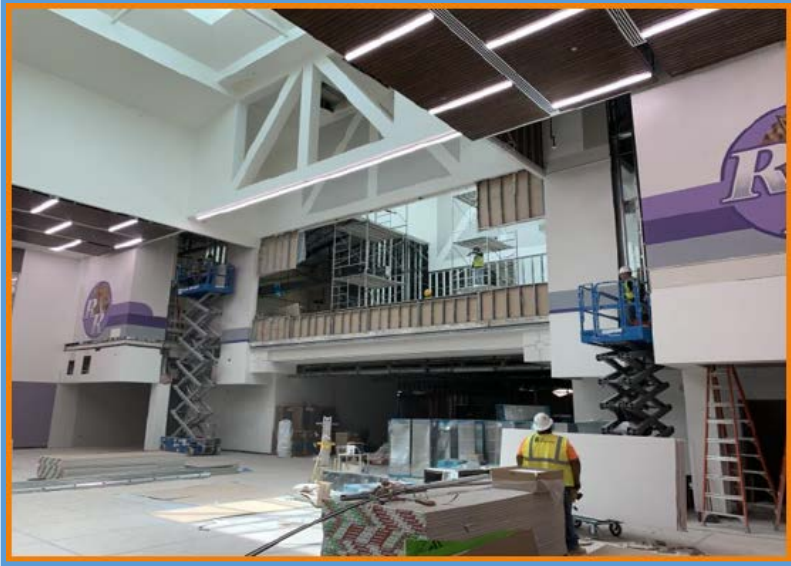
Robinson Middle School, Wood Ceiling in Cafeteria, July 2019
