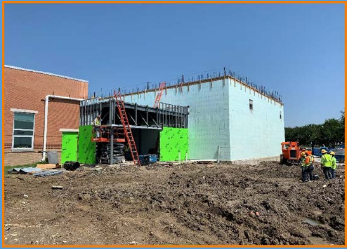
Rice Middle School Fine Arts Addition, Band Hall and Corridor Addition, July 2019
