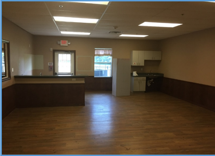
Employee Child Care 3, Interior Rooms under Construction, June 2018
