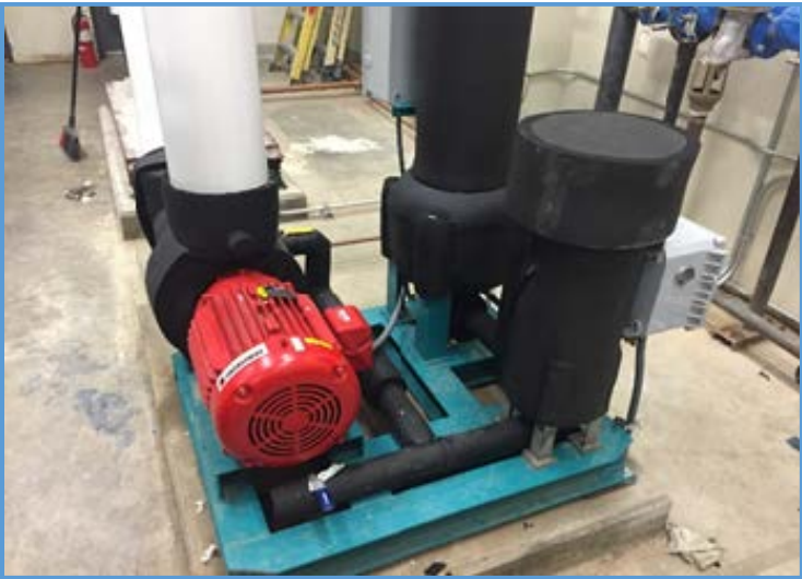
Gulledge Elementary School, New Soils Separator, September 2018
