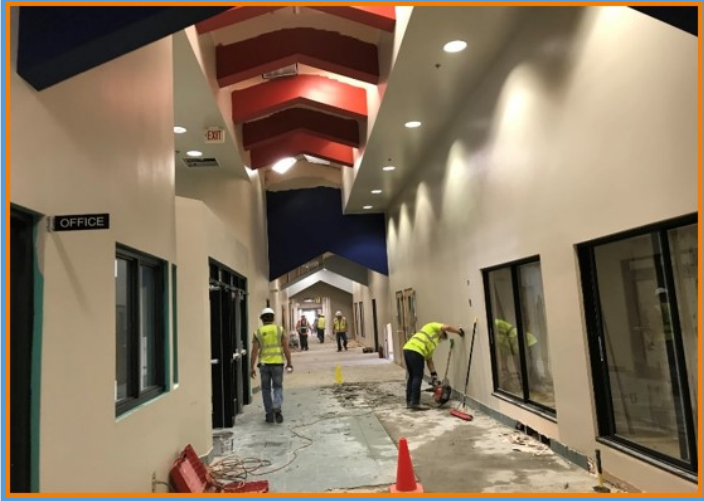
Skaggs Elementary School, Main Street Demo, July 2019
