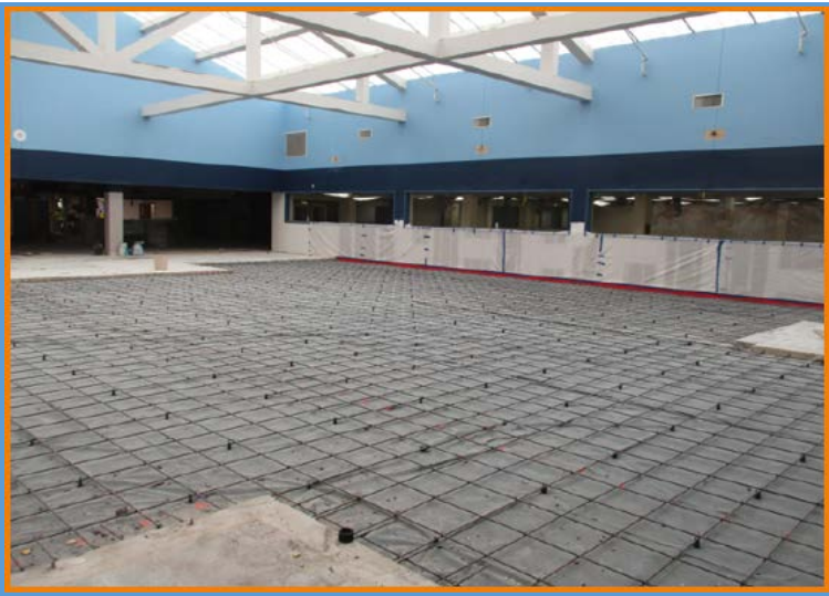
Bowman Middle School, Student Commons Concrete Infill, July 2019
