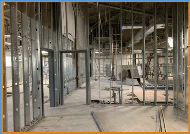
Robinson Middle School, Stud Framing in 2 nd Floor Science, July 2019
