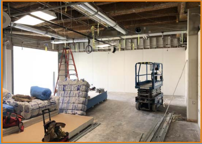
Vines High School Art Renovation, Sheetrock in CTE Suite, July 2019
