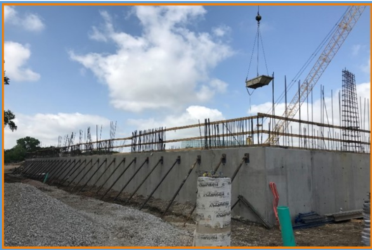
Fine Arts Center, Below Grade Walls at Studio Theater, July 2019
