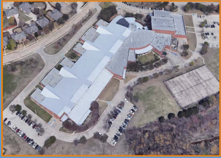
Frankford Middle School Fine Arts Addition, Aerial of Site, July 2019
