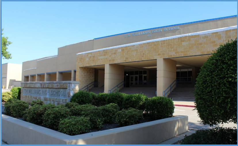
Williams High School, Main Entry, June 2018
