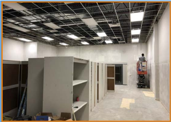
Armstrong Middle School Fine Arts Addition, Demo in Existing Fine Arts Suite, July 2019
