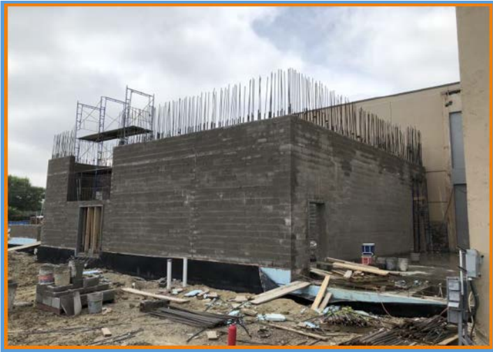
Armstrong Middle School Fine Arts Addition, CMU Block Wall Installation, July 2019
