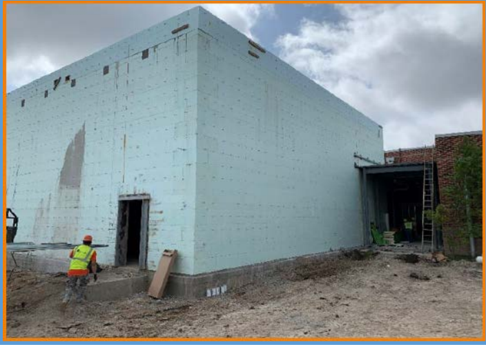
Renner Middle School Fine Arts Addition, Band Hall Addition, July 2019
