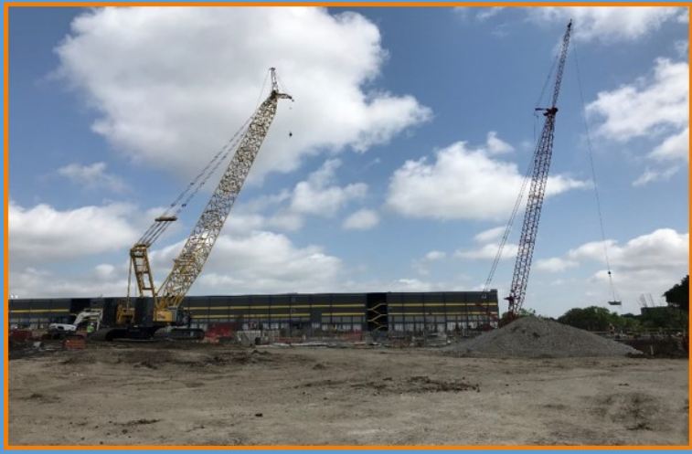
Fine Arts Center, Running Two Cranes as Walls Go Up, July 2019
